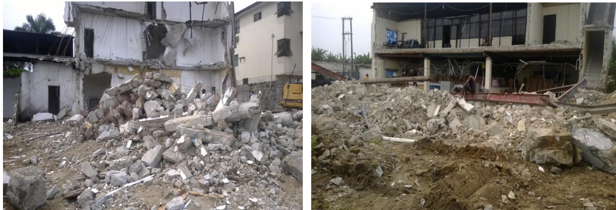
Figure 1: Concrete Demolition Waste along Trans-Amadi, Port Harcourt, Nigeria.
